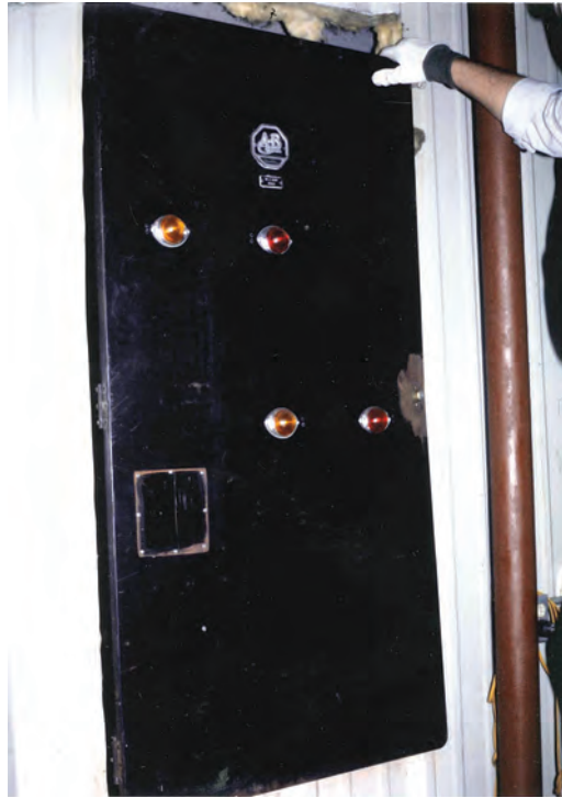
Figure 2. Electrical control panel used as a secret access door to the hidden storage rooms with tanks for liquid beet sugar.
