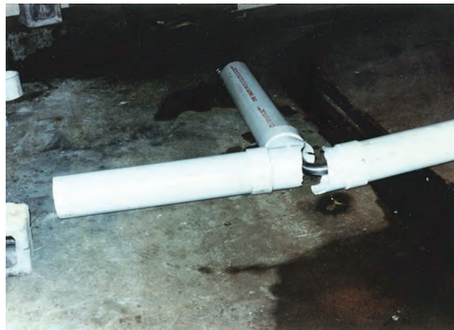
Figure 3. Hidden stainless steel pipe system used for moving liquid beet sugar from secret holding tanks to the processing line. The system was hidden inside a fake PVC drainage system.
